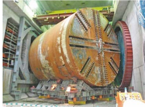
Photo 1 U-turning of shield machine
