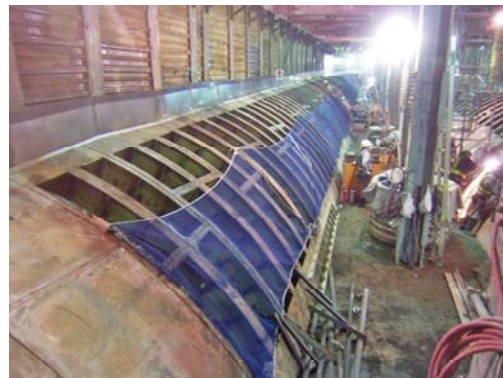
Photo 2 Enlargement of the space by cutting segments
