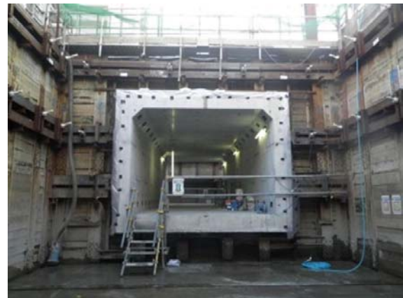
Photo 2 Completion of construction of precast box
