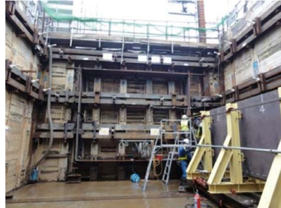
Photo 1 Insertion of protective steel plates
