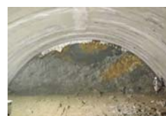
Photo 1 Tunnel face of upper half
