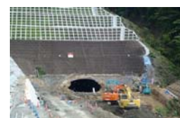
Photo 2 Penetration of tunnel portal with earthmoving
