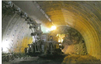
Photo 1 Tunnel excavation
