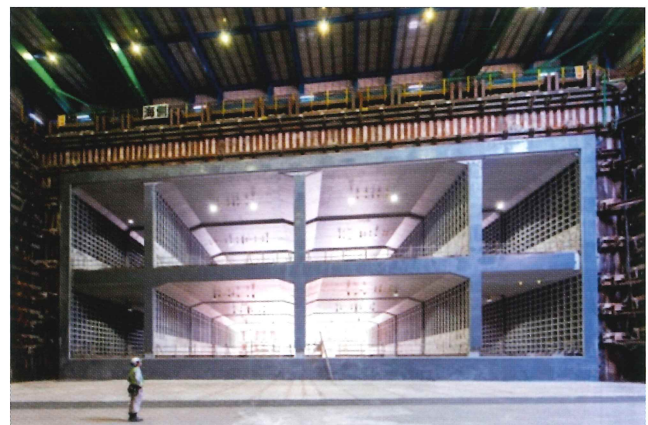
Fig. 3 Completion of the box culvert traction
