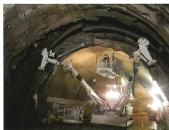
Photo 5 Reconstruction of a collapsed area
