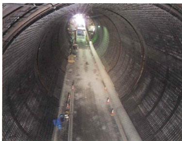
Photo 2 Completion of the reinforcement
