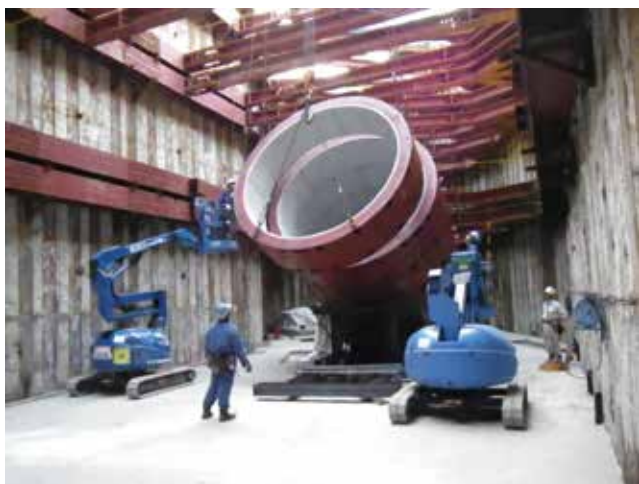
Photo 2 Assembly situation of composite segment rings
