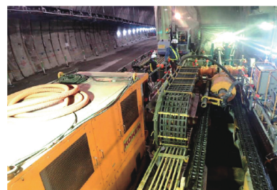
Fig.2 Construction with the FSC-100
