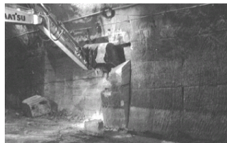
Hydraulic splitting work in the tunnel 25 June 2011
