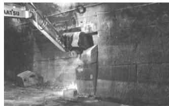
Hydraulic splitting work in the tunnel 25 June 2011
