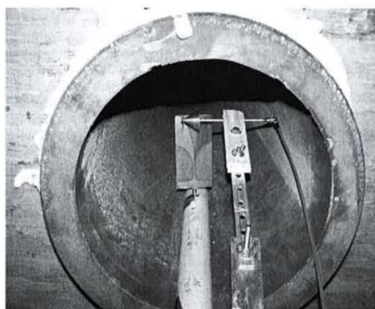
Fig. 9. Arrangement of antennas inside a 0.30 m clay pipe with Vivaldi antenna positioned in the vertical direction and the disccone antenna aligned in the horizontal direction.
