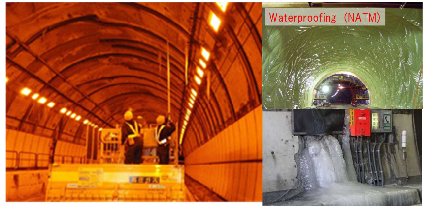
Water Leakage and freezing (icicles)
