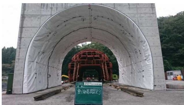
Installation of waterproofing
