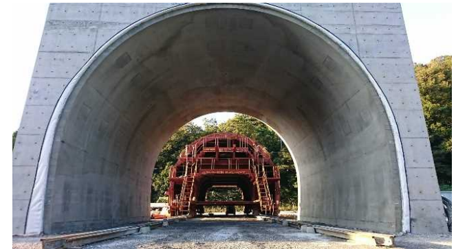
Lining concrete placement
