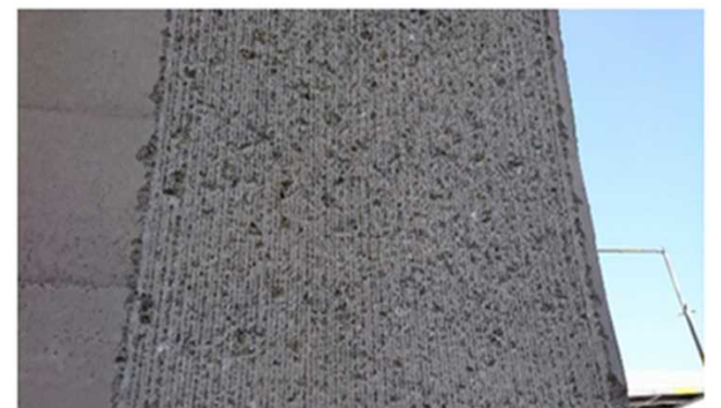
Cutting lining concrete
