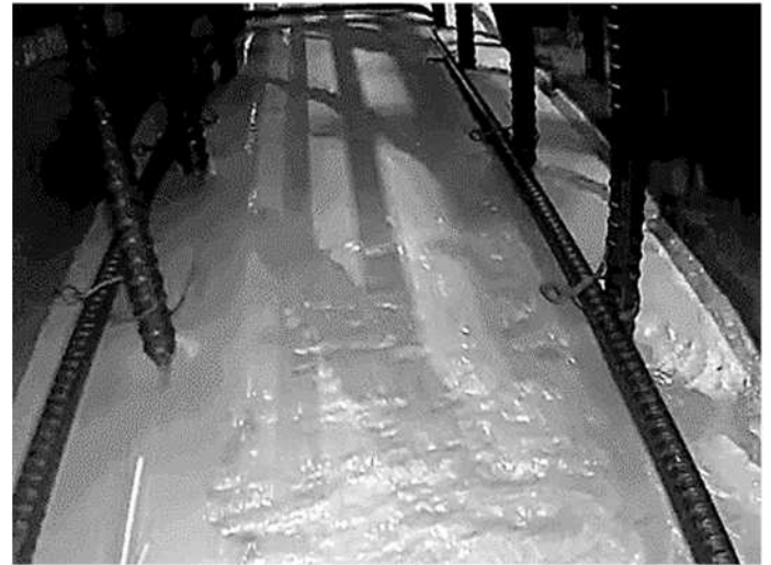
Picture-4 Situation of SCC pressurized filling
