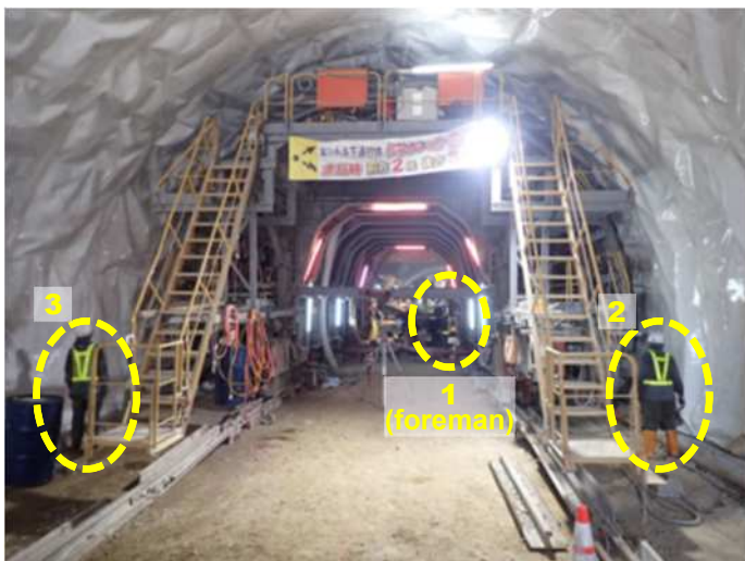
Picture-6 Situation of Filling Concrete (Conducted by only 3 workers)
