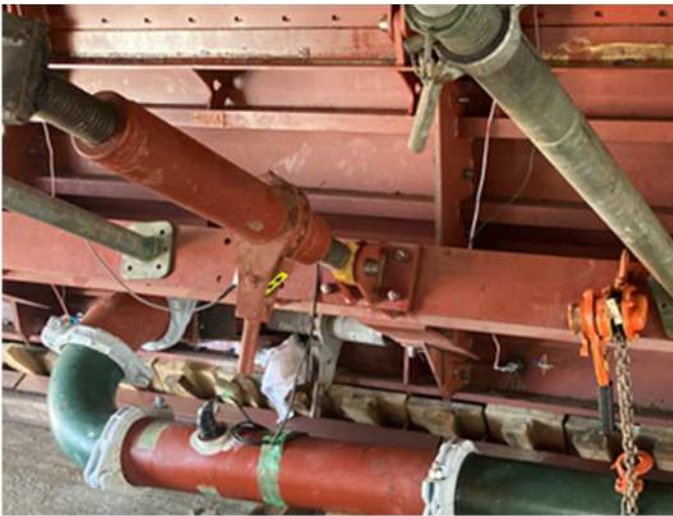
Picture-3 Injection slot
