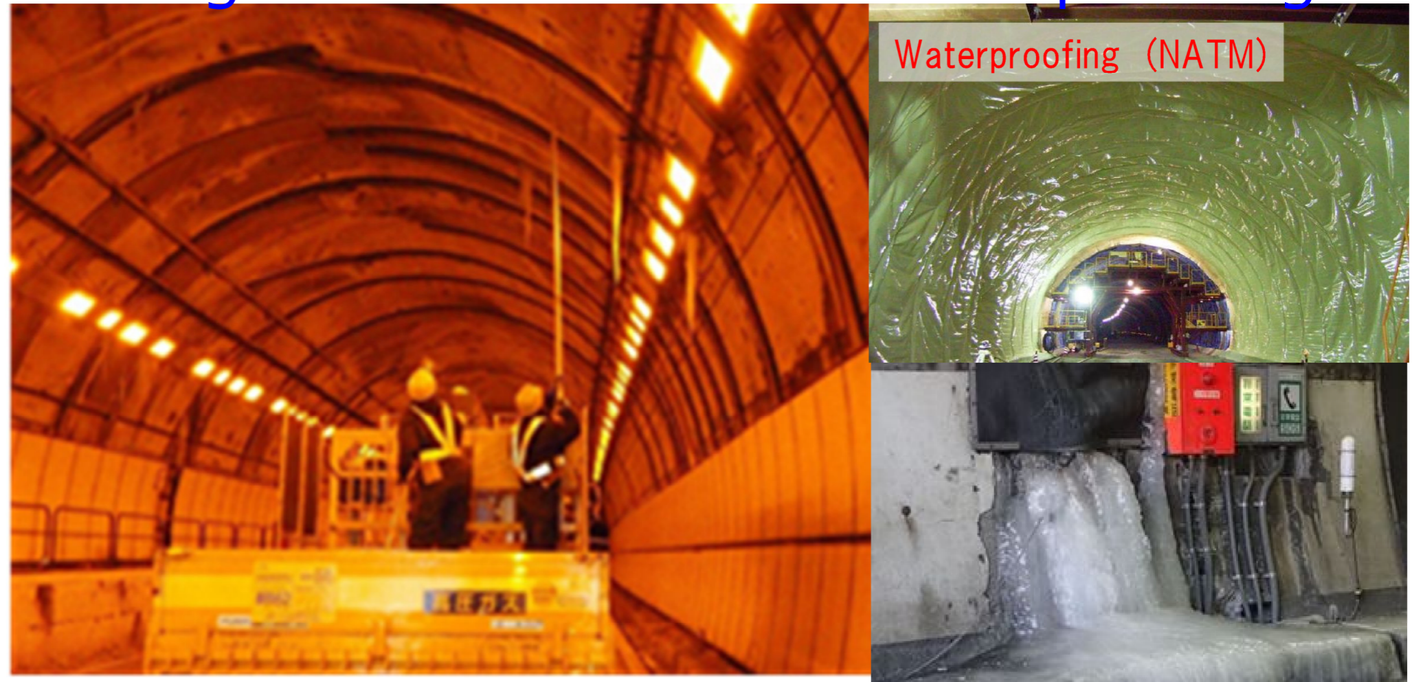
Leakage and Its freezing (icicles)
