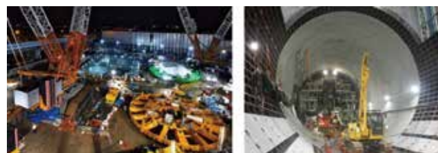
Fig. 4 Assembling of the cutter and view inside the tunnel
