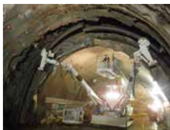
Photo 5 Reconstruction of a collapsed area
