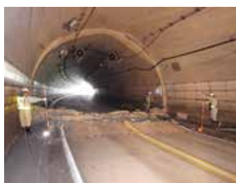
Photo 2 Compressive destruction and earth heaving
