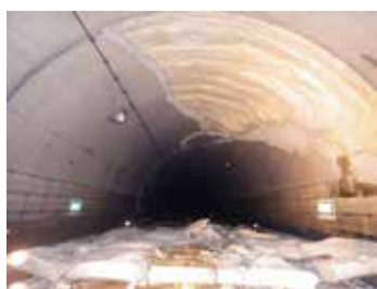
Photo 1 Collapse of lining concrete
