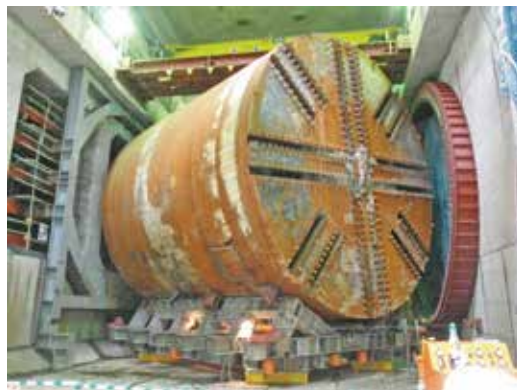
Photo 1 U-turning of shield machine
