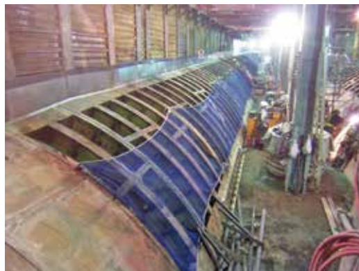
Photo 2 Enlargement of the space by cutting segments
