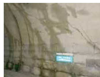
Photo 3 Openings and cracks caused by shearing force
