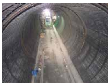
Photo 2 Completion of the reinforcement
