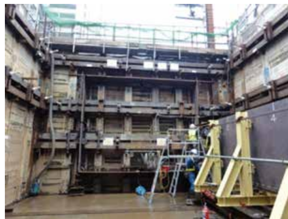
Photo 1 Insertion of protective steel plates
