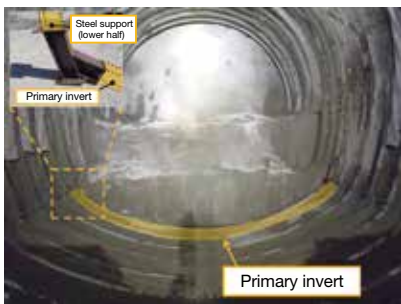
Fig. 1 Construction of primary inverts
