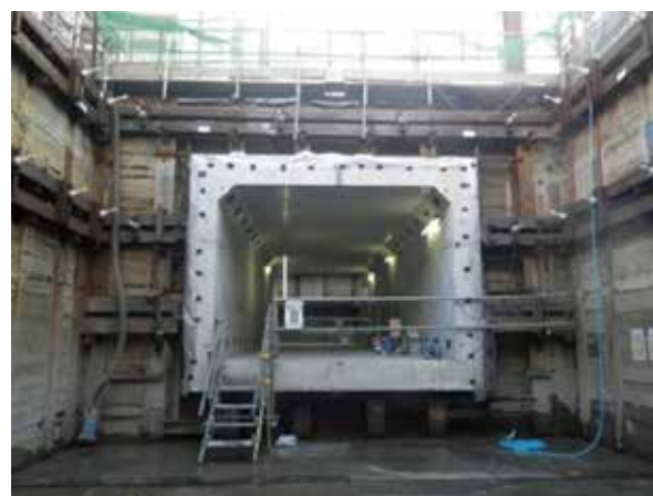
Photo 2 Completion of construction of precast box
