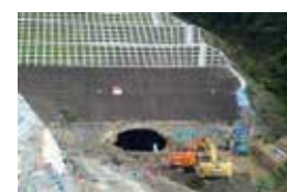
Photo 2 Penetration of tunnel portal with earthmoving
