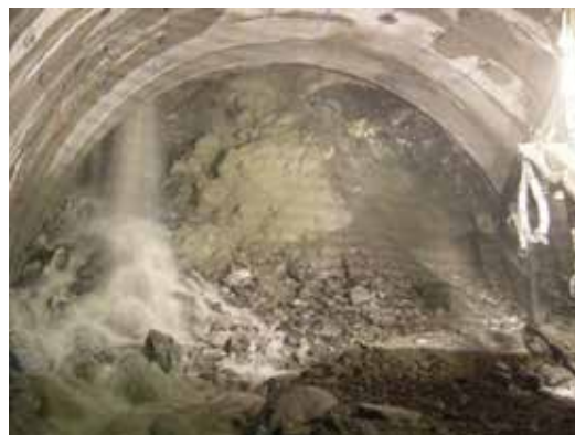
Photo 1 Water gush during tunnel excavation
