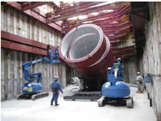
Photo 2 Assembly situation of composite segment rings
