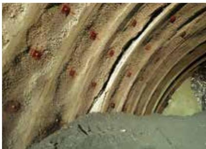
Photo 1 Extrusion of primary support
