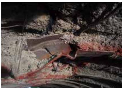
Photo 2 Buckling of steel support
