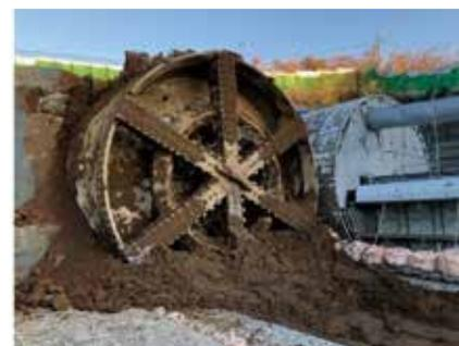
Fig. 4 A tunnel reaching aboveground
