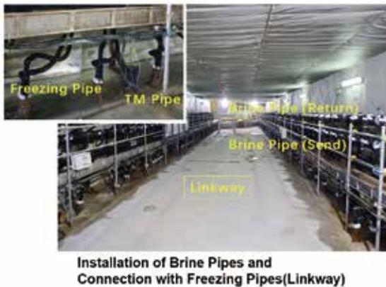
Fig. 1 Freezing Pipes
