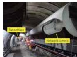
Fig. 2 Installed network camera
