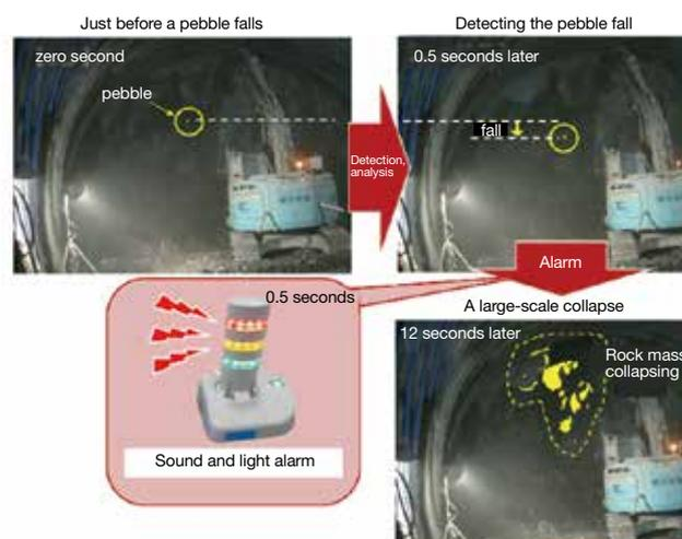
Fig.2 Rockfall detection using moving image during excavation
