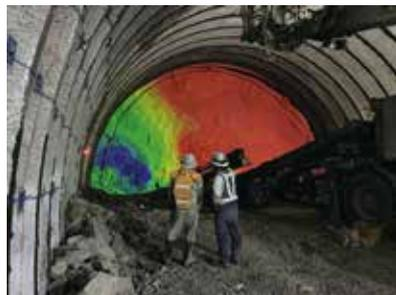
Photo 1 Projection of a Drill Hole Energy Contour Diagram
