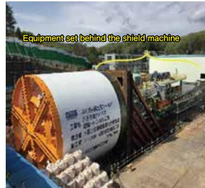
Fig. 2 Equipment set and launching at ground level
