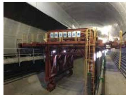
Fig. 3 Bogie-type internal support
