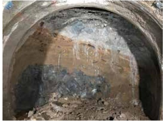
Photo-2.1 A Tunnel Face Sample in Japan with Soft and Hard Ground
