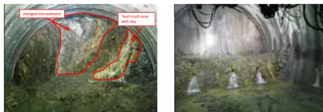
Fig. 2 Condition of the Fault Crush Zone during Excavation
