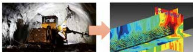
Drilling by auto-controlled face drilling rig      Prediction by ordinary kriging
