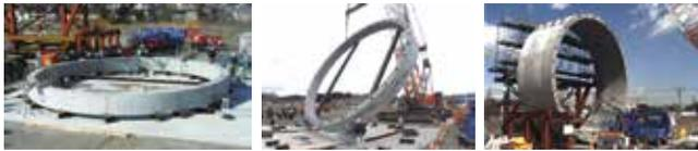
Photo 1 Assembly of segments above ground
