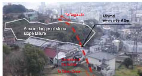
Fig. 1 Surface Condition of Area A
