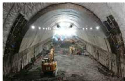
Photo 1 Bench excavation, 3<sup>rd</sup> stage
