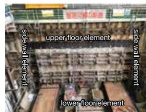
Photo 3 launching shaft (lower floor element drilling)
