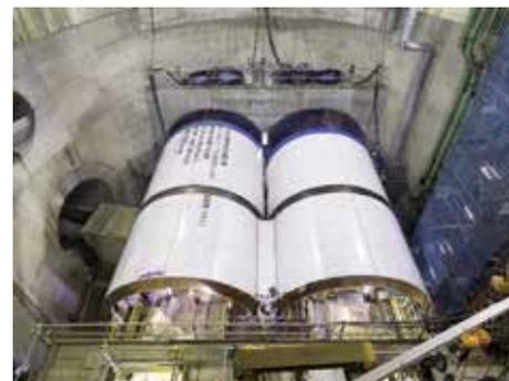
Fig. 3 H&V shield machines in vertical shaft
