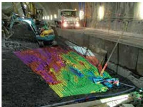
Photo 1 Projected image on the excavation area
