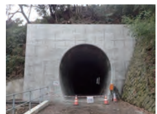
Photo 4 Portal restoration conditions
