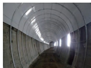
Photo 3 Inner reinforcing by T3 panel method
