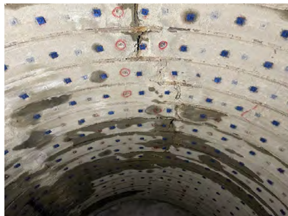
Photo 1 Damage of support members at large earth pressure area
