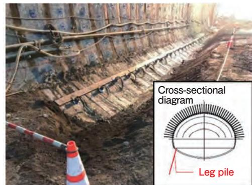
Fig. 4 Construction of leg piles
