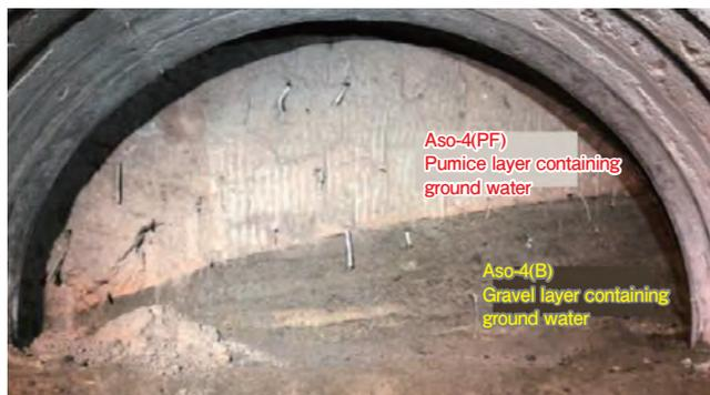
Fig. 2 Geological conditions of the face in the section where the deformation occurred
