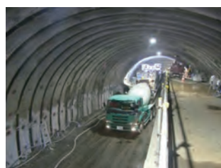
Photo 2 Concrete spraying (under tunnel ventilation)
