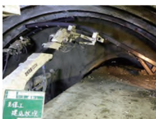
Photo 1 Installation of the tunnel support
