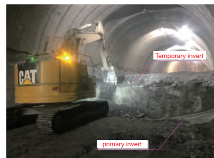
Photo 1 The temporary invert
