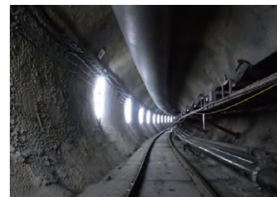
Photo 3 Full view inside the TBM tunnel (support type B1)
