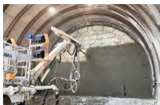
Fig. 2 Automated shotcreting machine
