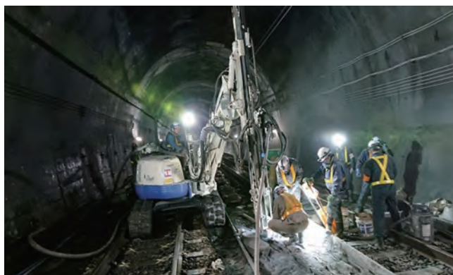
Photo 1 Self-drilled rock bolt placing
