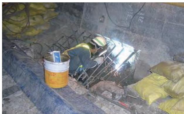
Photo 2 No-shrink mortar placing
