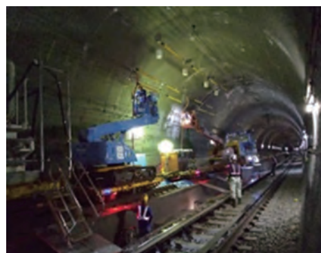
Photo 1 Injection behind the lining
