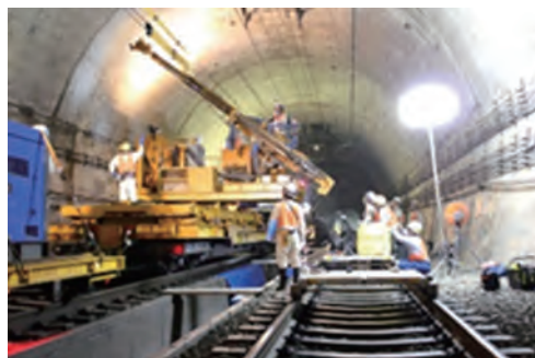
Photo 2 Rock bolt installation
