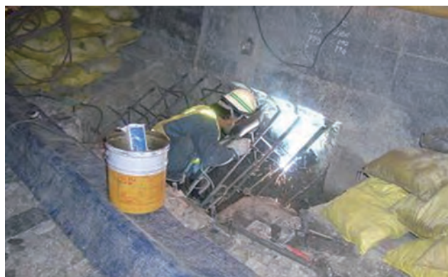
Photo 2 No-shrink mortar placing
