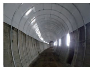
Photo 3 Inner reinforcing by T3 panel method
