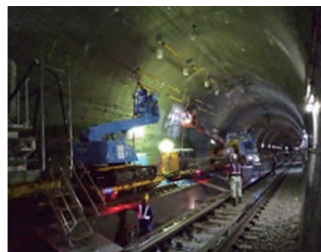
Photo 1 Injection behind the lining
