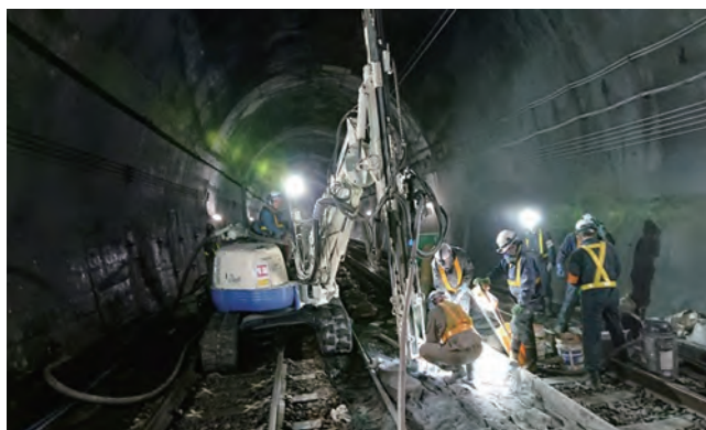
Photo 1 Self-drilled rock bolt placing
