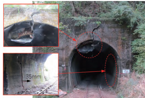
Photo 2 Lining deformed conditions
