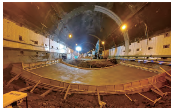
Photo 1 After placing invert concrete
