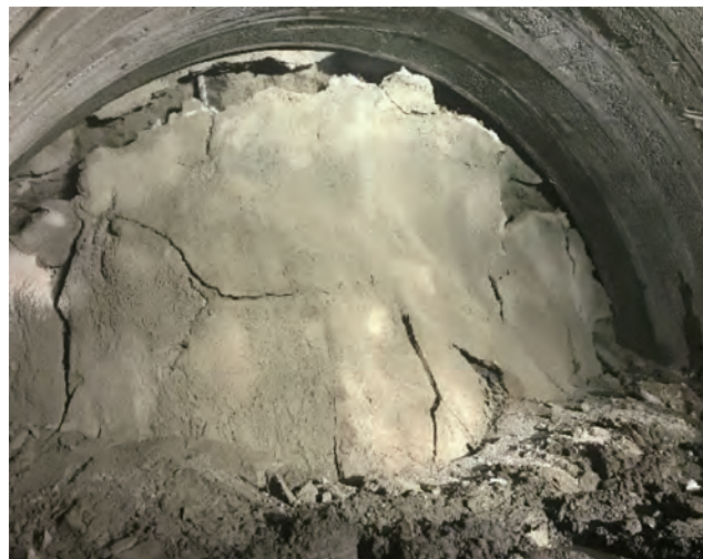
Photo 2 Ground squeeze
