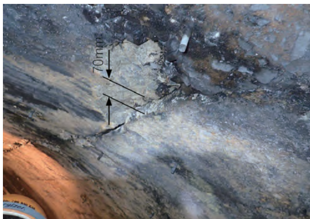
Photo 1 Portal deformed conditions
