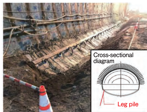
Fig. 4 Construction of leg piles
