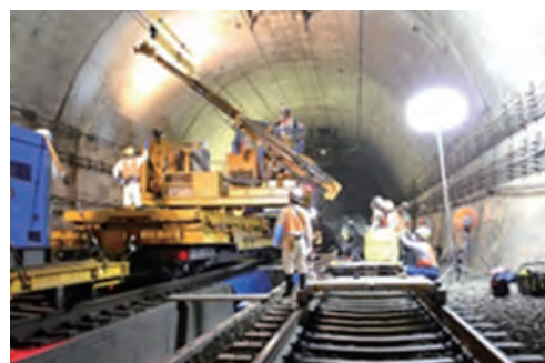
Photo 2 Rock bolt installation
