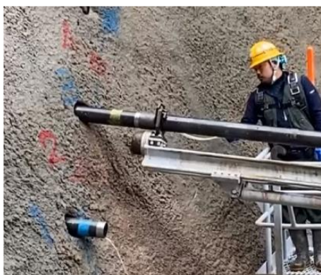
Illustration of a socket-type connection with simple plug-in installation
