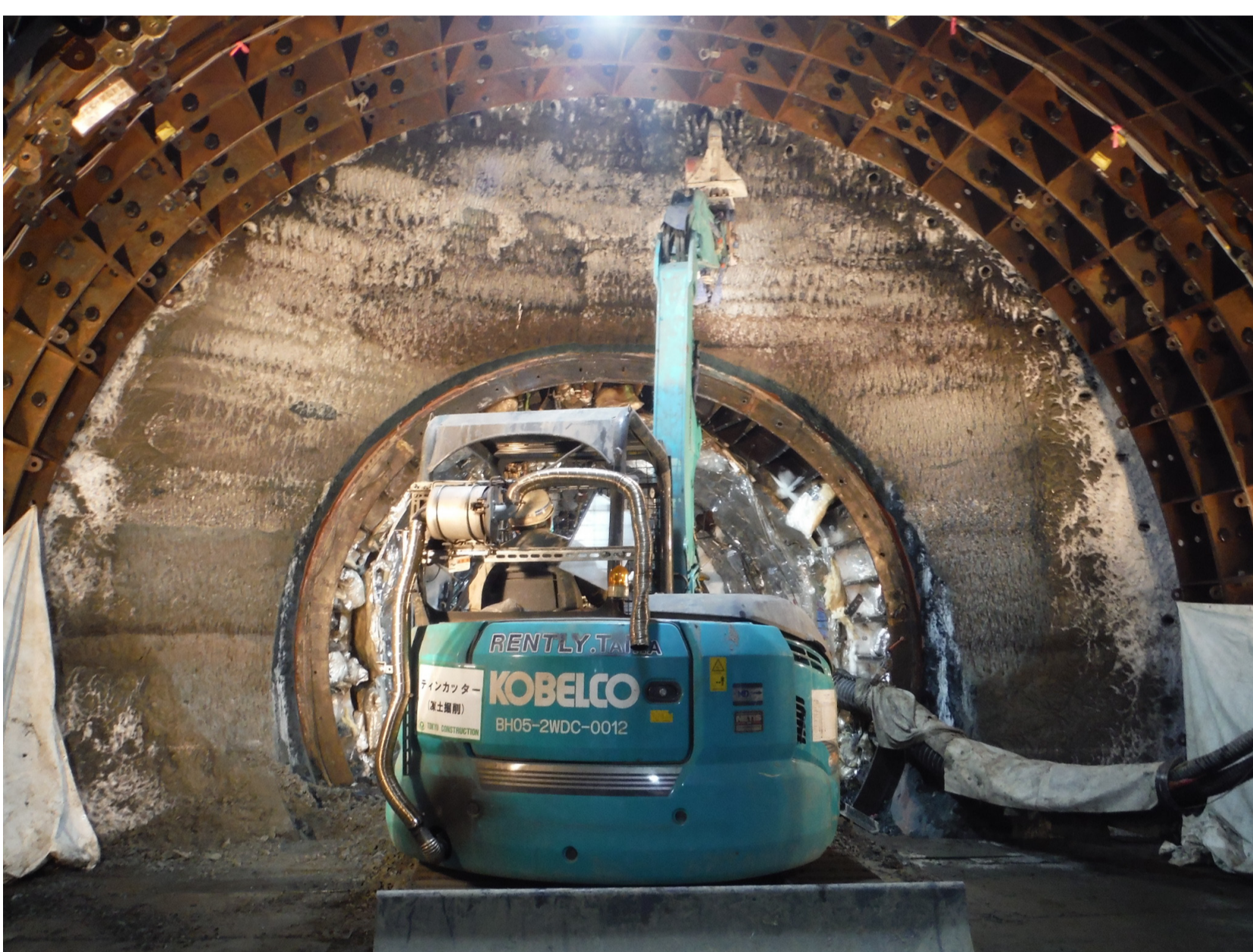
2. Excavation of Frozen Soil
