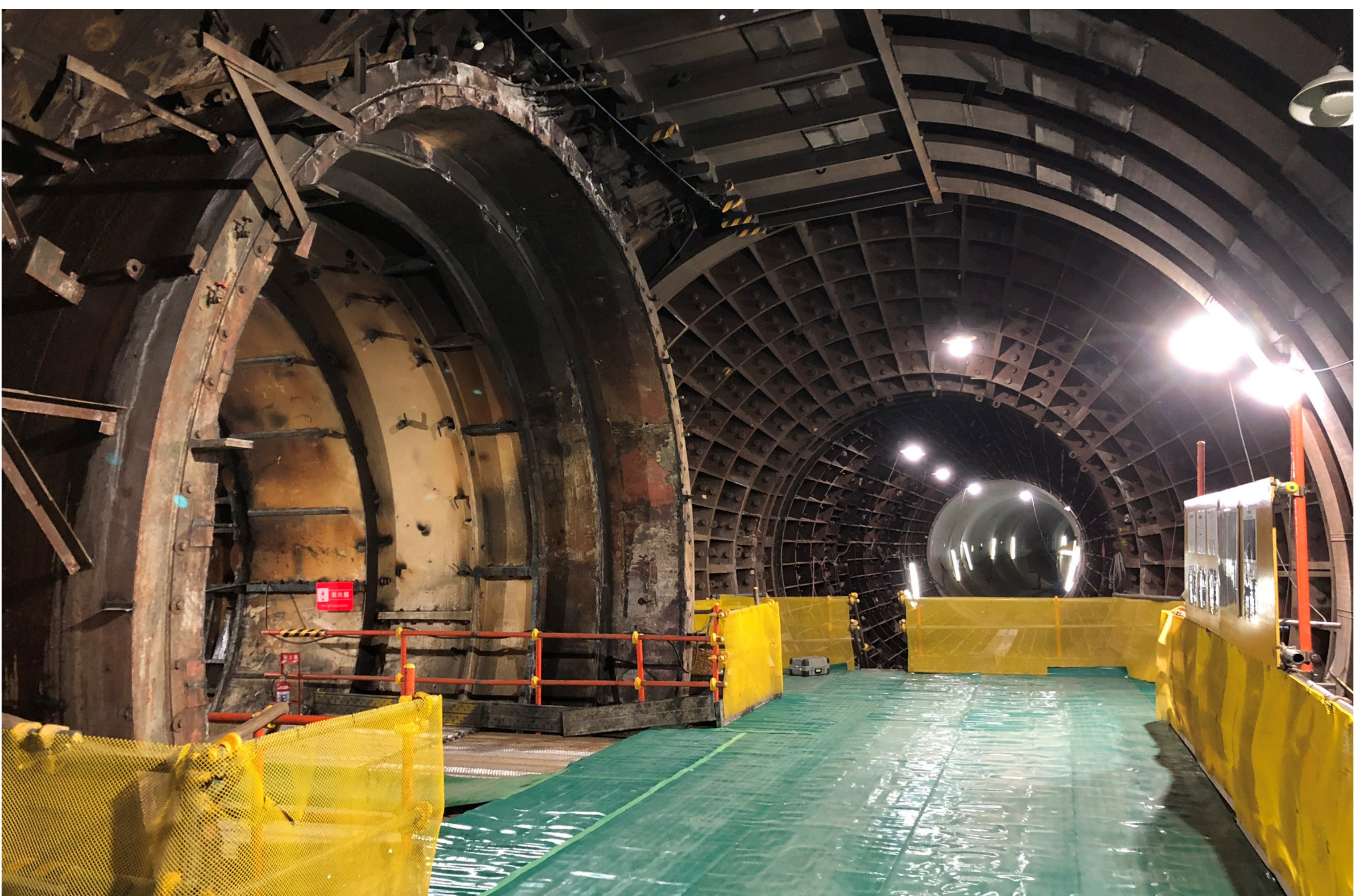
6. Completion of Connection
