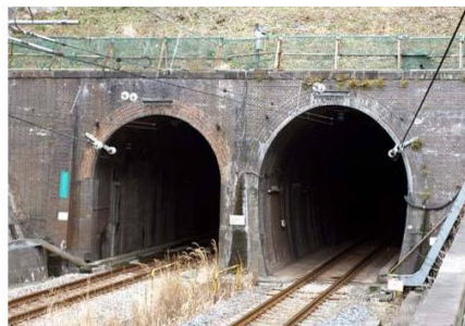
Fig. 2 Legacy Tunnel (Left side tunnel), approximately 140 years in service
