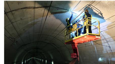
Fig. 3 Close inspection of tunnel linings by in-house engineers
