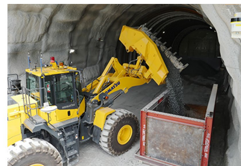
Automated wheel loader in the mock-up tunnel
