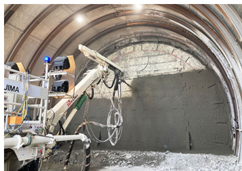
Automated shotcreting machine in the mock-up tunnel
