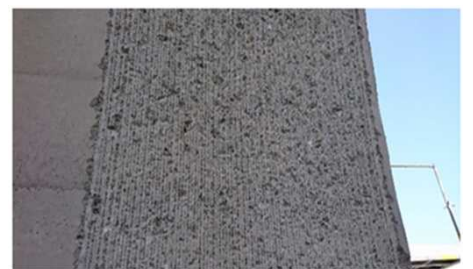
Cutting lining concrete
