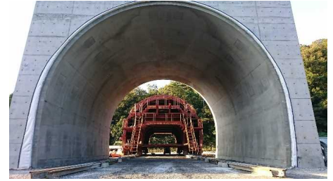
Lining concrete placement
