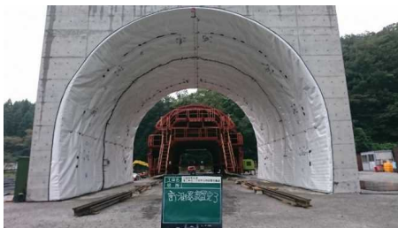
Installation of waterproofing
