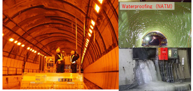
Water Leakage and freezing (icicles)
