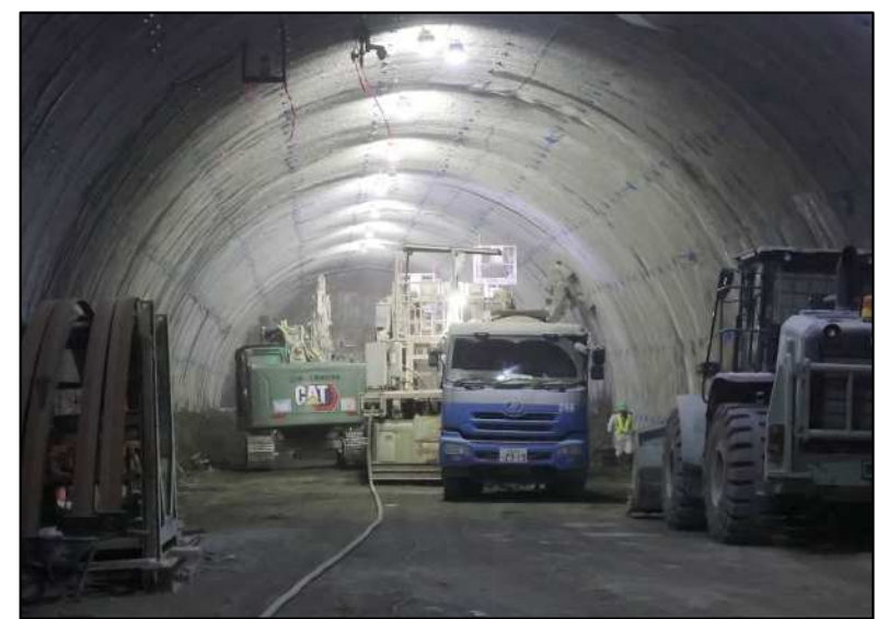
H-Rampway Section (As of December 2023)
