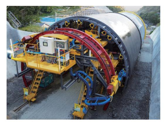
The system has the capability to automate concrete pouring, compaction, and stop-pouring operations fully. A blow-upward pouring method with flowable concrete is utilized to ensure consistent and uniform concrete quality.
