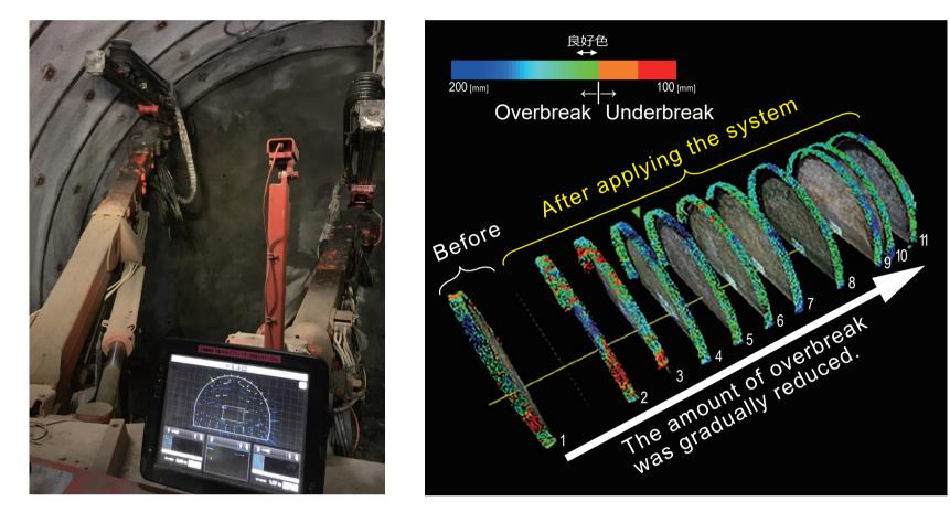
The system is designed to automatically control the insertion angle of the outermost circumference holes during blasting. This can help reduce overbreak and underbreak, improving productivity and safety. Furthermore, this system does not require skilled workers.
