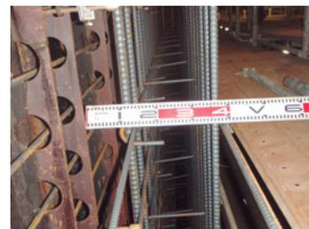
Fig. 5 Assembled PBL and side wall reinforcement
