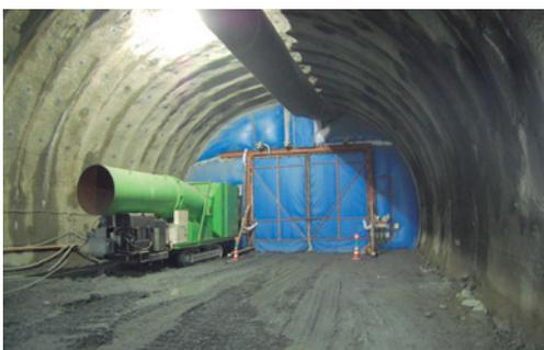
Fig. 2 Electrostatic precipitator and movable balloon bulkhead (view from the portal side)
