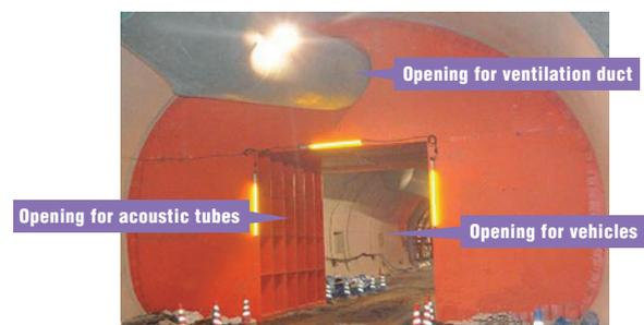
Fig. 1 Blast Silencer® installed
