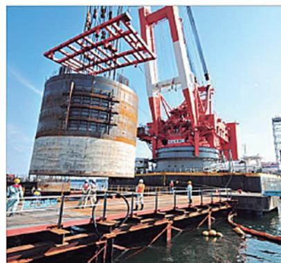
Photo 1 Placement of a caisson's cutter unit
