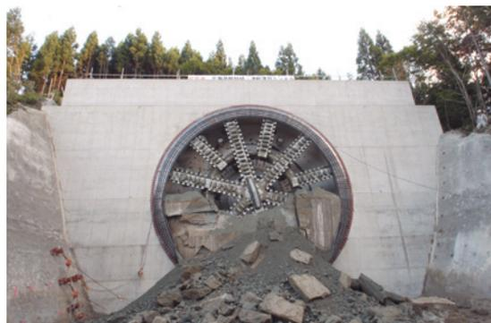
Photo 1 SENS's breakthrough to the portal
