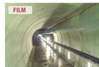
Photo 1 Installation of waterproofing membrane
