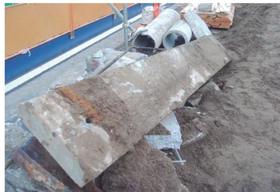
Photo 2 Debris remaining in the reclaimed ground
