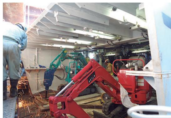
Photo 3 Open type shield machine
