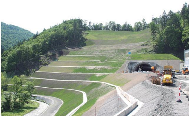
Photo 1 Landslide prevention
