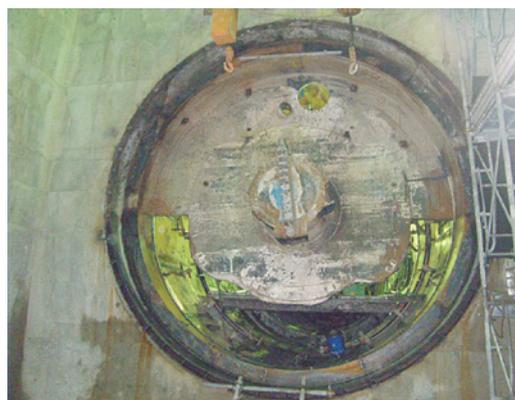
Photo 2 After dismantling of the face plate
