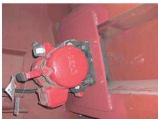
Photo 1 Form vibrator installed
