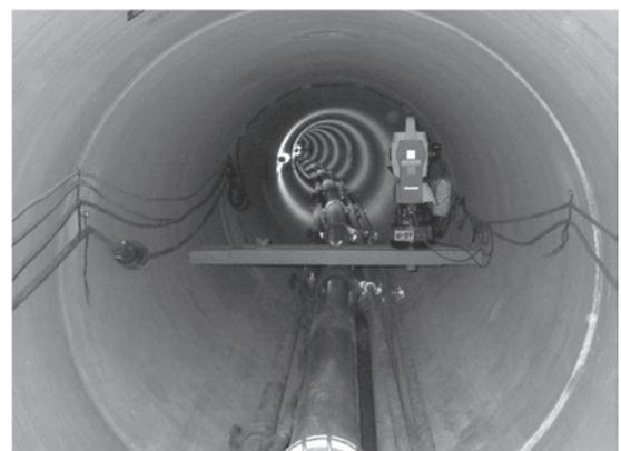
Photo 2 Installation of automatic survey equipment
