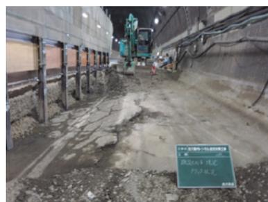
Photo 2 Damage of the old invert
