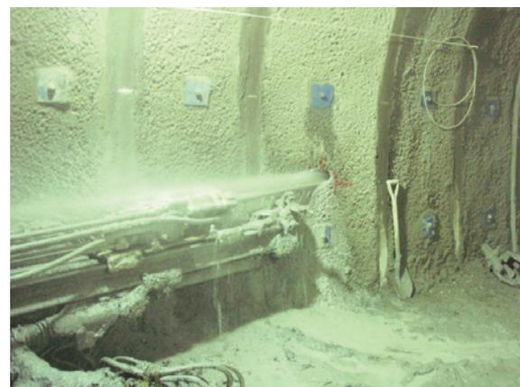
Photo 3 Methane gas blasting out
