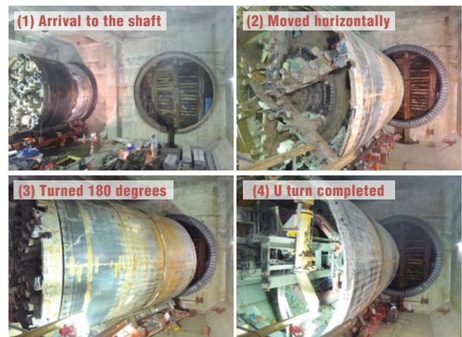
Photo 2 U turn process of the machine
