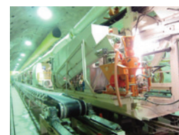
Photo 2 Fiber mortar spraying equipment mounted on TBM
