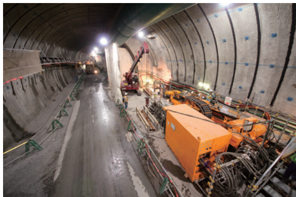
Photo 1 1,000 m-class ultra-long pilot boring
