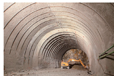
Photo 2 Smoothing of shotcrete surface (up front: WT section, in the back: non-WT section)
