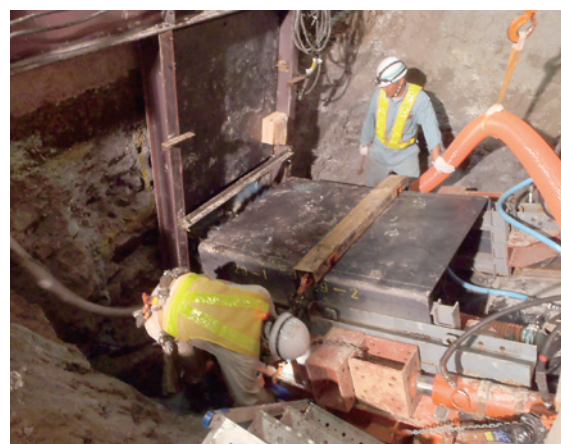
Photo 2 View of the box in place (placement of the steel box)
