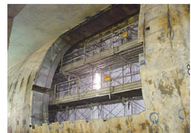
Photo 2 Segment cutting (work side)
