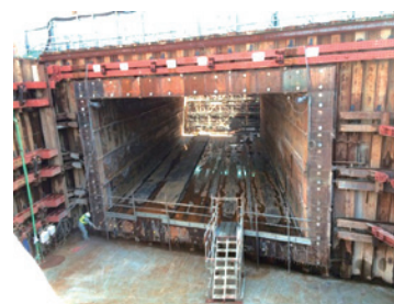
Photo 2 Box culvert
