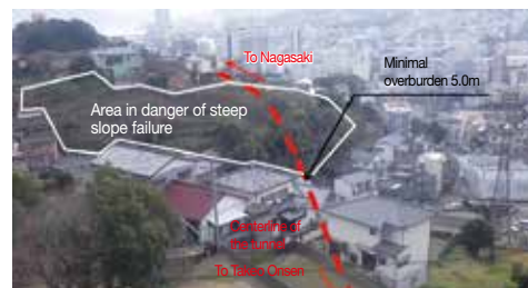
Fig. 1 Surface Condition of Area A
