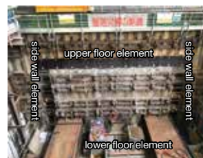
Photo 3 launching shaft (lower floor element drilling)
