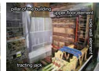
Photo 4 Arrival shaft (drilling the side wall element)
