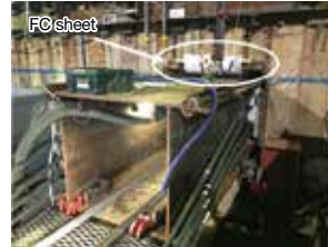
Photo 2 FC sheet (standard element 1080mm x 850mm)
