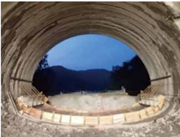
Photo 1 Largest Excavation Section with size 226m 2
