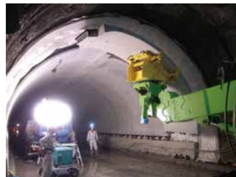
Fig. 2 Construction in progress
