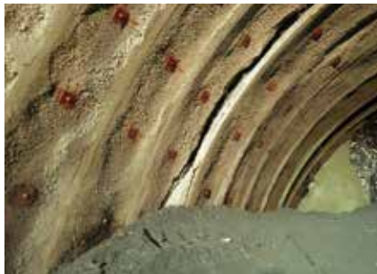
Photo 1 Extrusion of primary support
