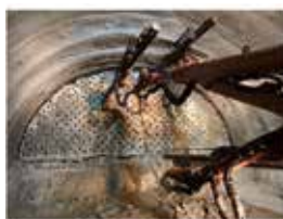
Photo 1 Work of Continuous Holes and Rock Breaking Hole
