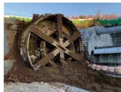
Fig. 4 A tunnel reaching aboveground
