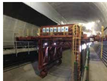
Fig. 3 Bogie-type internal support
