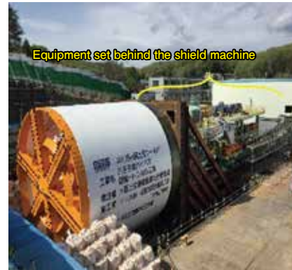
Fig. 2 Equipment set and launching at ground level
