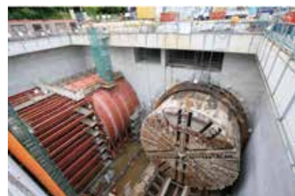
Photo 2 Arrival of the Shield
