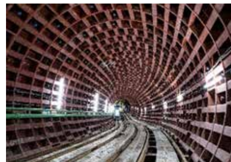
Fig. 4 Inside photo of the spiral drilling section
