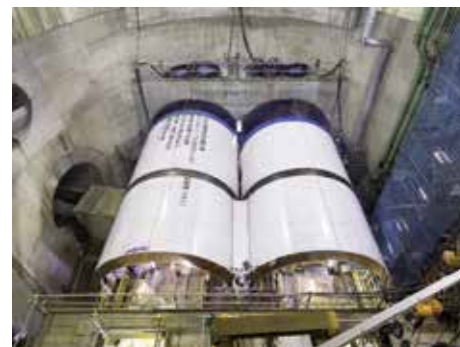
Fig. 3 H&V shield machines in vertical shaft
