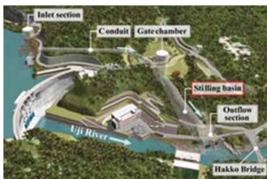
Fig. 1 Layout of tunnel-type discharge facility
