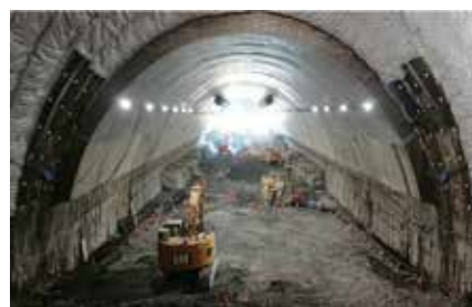
Photo 1 Bench excavation, 3 rd stage
