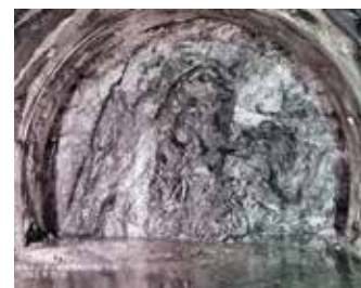
Photo Survey point No.37+82 Heavily folded cutting face
