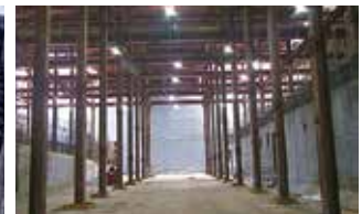
Fig. 5 Rationalization of temporary structures
