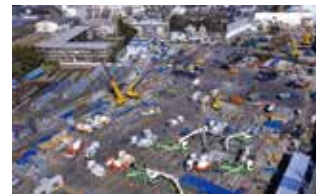
Fig. 4 Securing the work area through full lining
