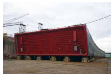
Photo 1 Steel shell of Tunnel element
