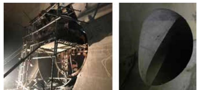
Photo 2 Underground connection complete
